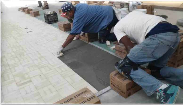
Treme Center Gym/Pool Repairs
